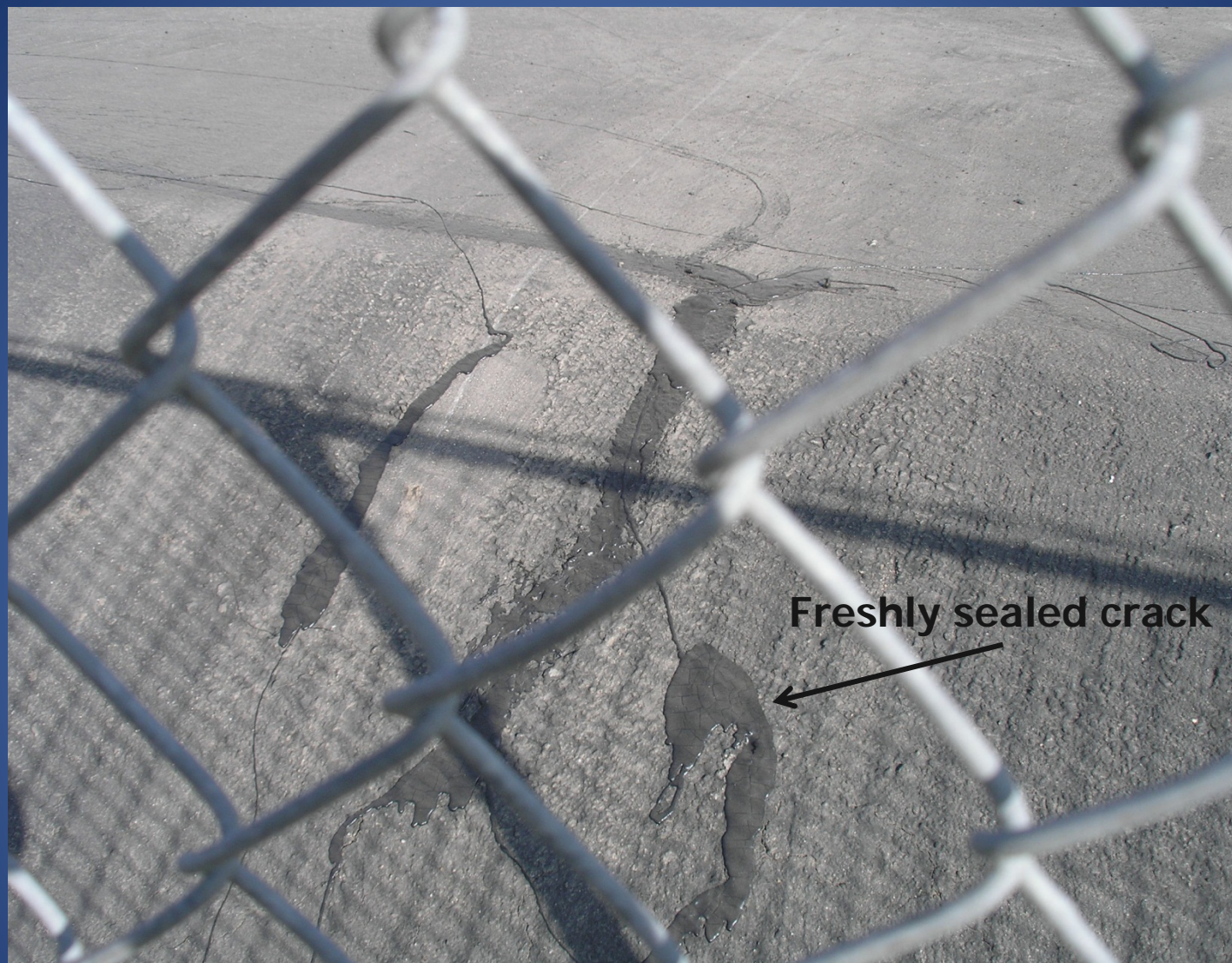
Picture taken through the fence at the edge of the asphaltic cap showing the freshly sealed cracks as dark areas on the cap. The repairs of the cap were required by the US EPA and were made in December 2011
