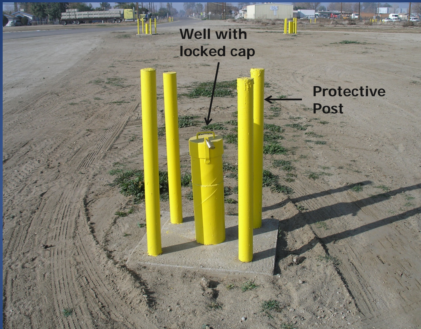
Off-site monitoring well from which groundwater samples are collected. Monitoring well has a locked cap and is surrounded by four protective posts. The locations of the current monitoring wells are shown in subsequent map from US ACE 3 rd 5-yr Review Report.
