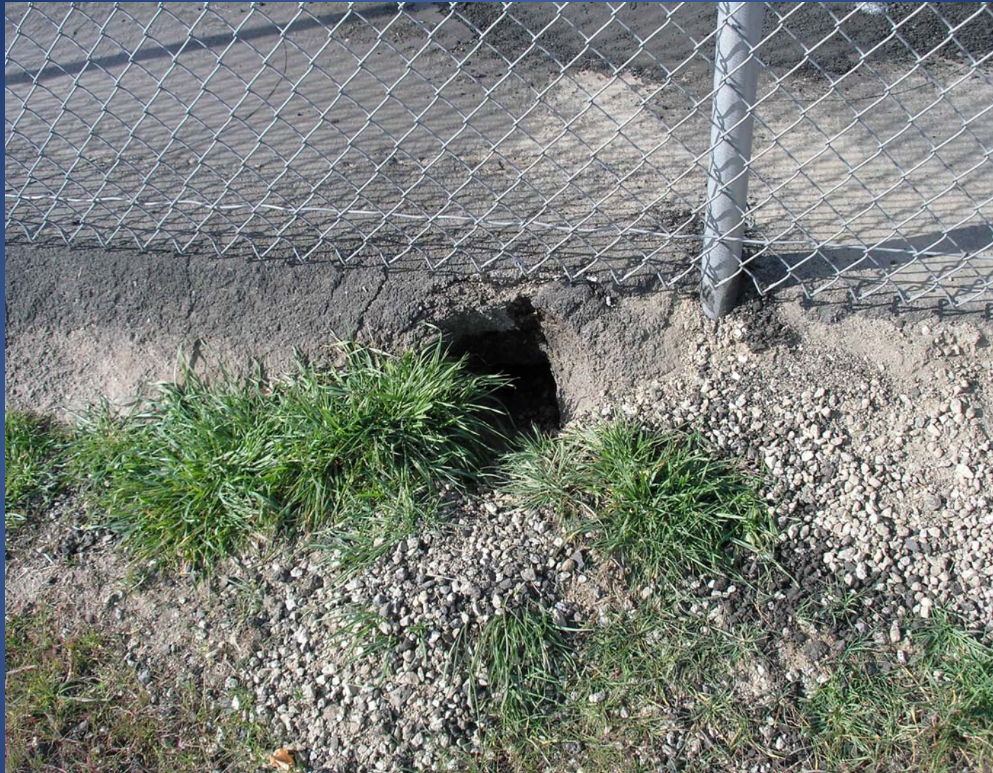
Large animal burrow that penetrates under the asphaltic cap.
