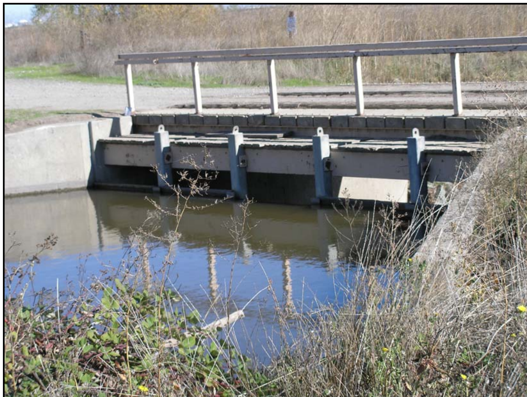
Figure 10. Los Rios Check Dam at the End of Putah Creek in the Yolo Bypass
