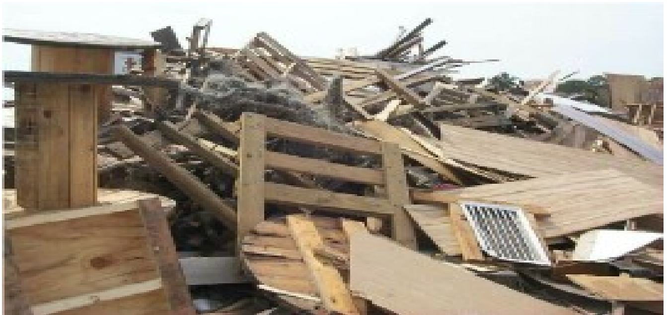
Demolition Debris with Possible CCA Treated Wood
